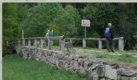
Stone bridge over the Malše and the state border
