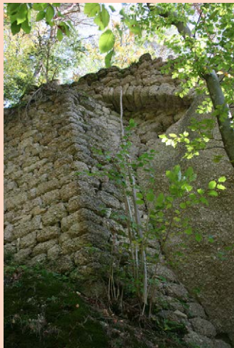
Wall remnants (left) and ring wall with relief arch (right)
